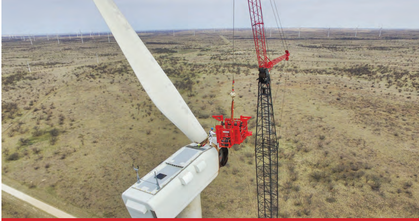
BIRD REMOVES BEARING FROM HUB
