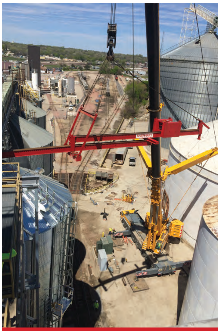
The Sioux City team uses a cantilever beam and counterweight with a 500-ton crane to install a 22,000 lb. tank at a plant.
