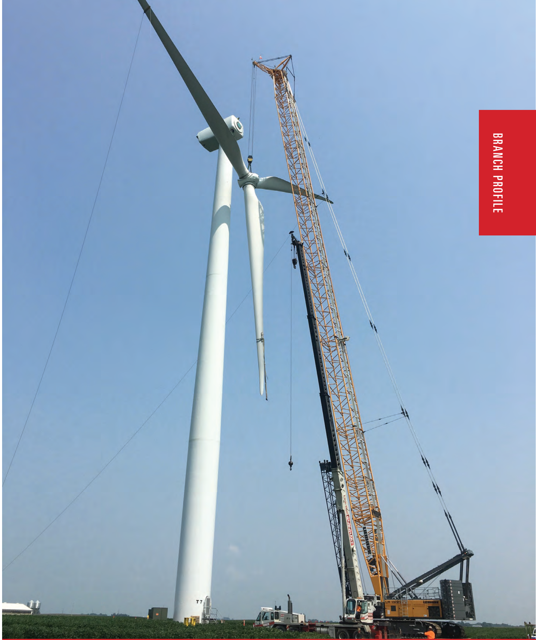
Barnhart uses their new LR1300SX to perform a gearbox replacement on an 80-meter tower in North Central Iowa.
